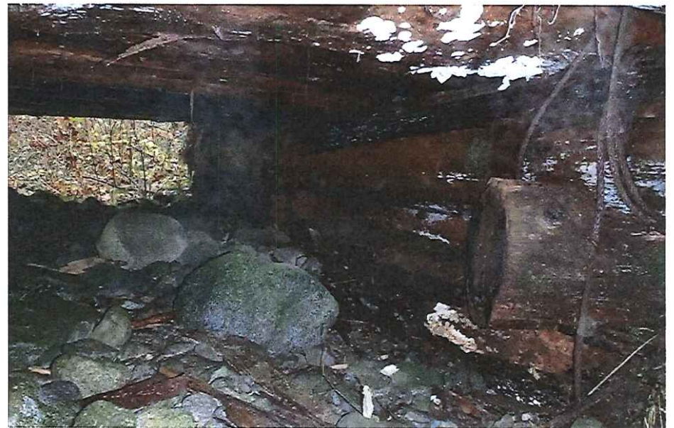
CK2266 Left Abutment
