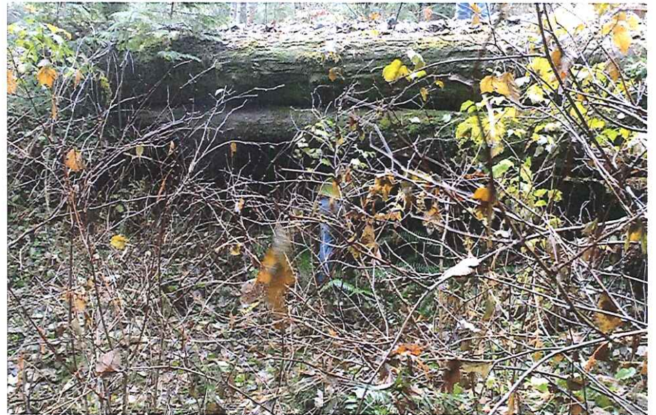
CK2266 From Downstream
