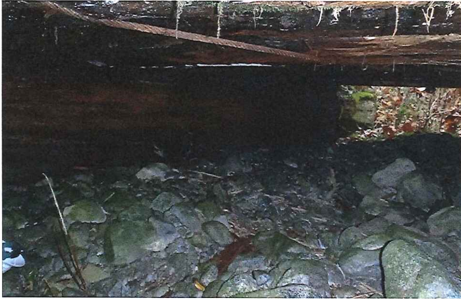
CK2266 Right Abutment
